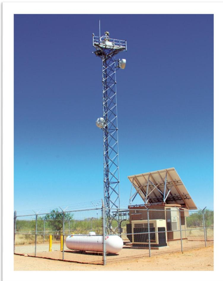
Pictured above is the integrated fixed tower system. This system consists of fixed towers, sensors (cameras and radar), a data communications network, facilities upgrades, information displays and an information management system. Initially developed as part of *SBI-Net*, numerous questions remain regarding the deployment of these technologies.
